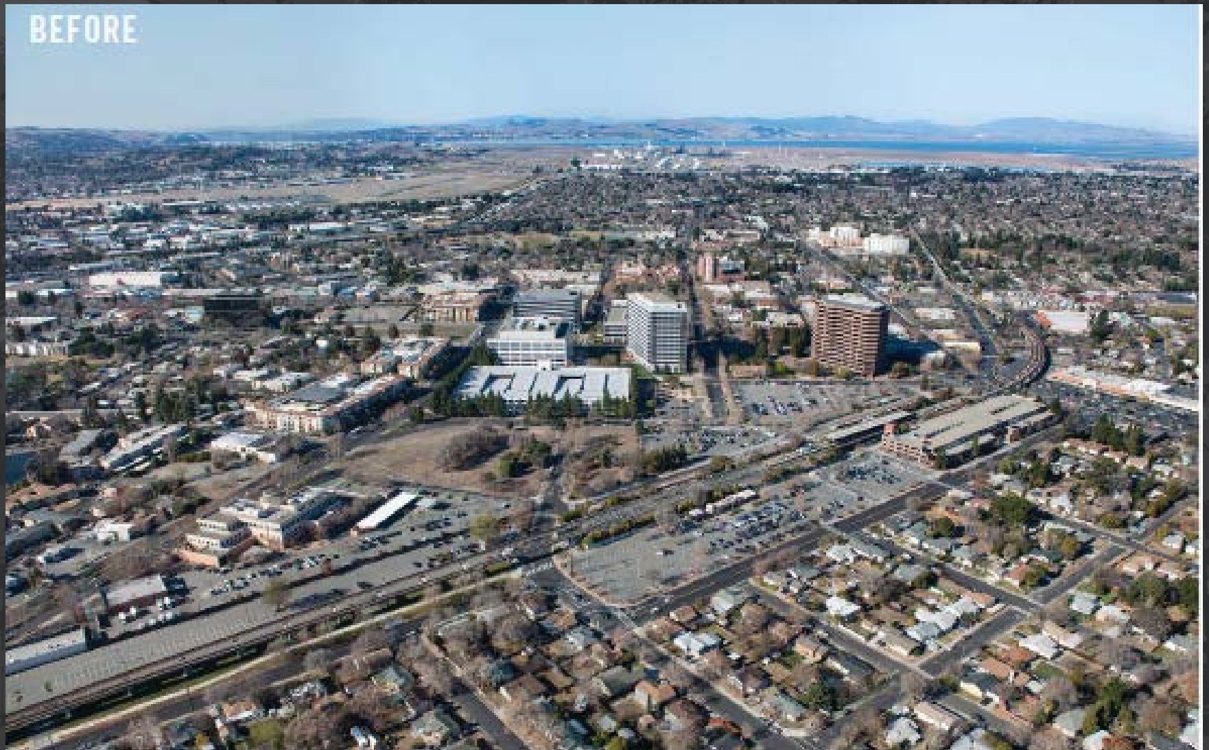
Existing Downtown Concord, looking north up Grant Street towards Todos Santos Plaza
